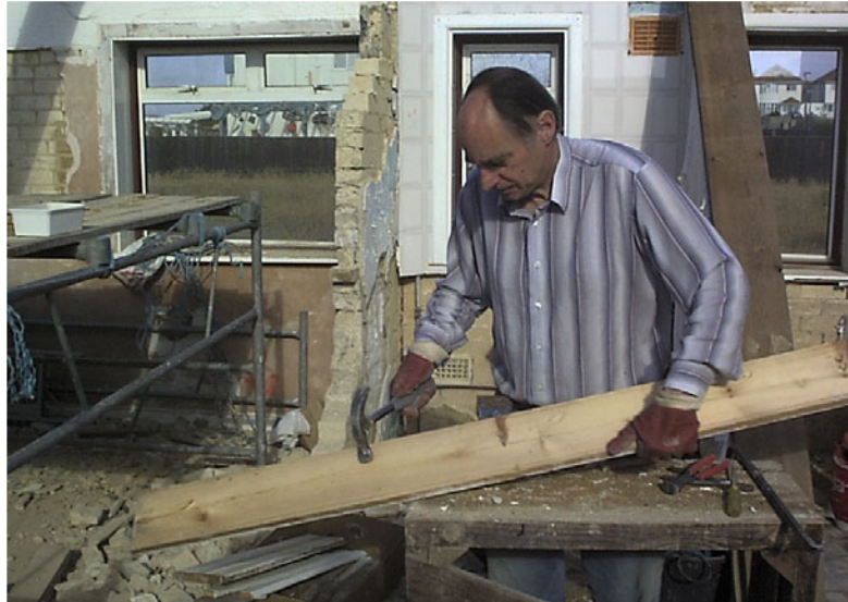
Doug de-nailing timber as part of his Master's thesis on sustainability and the recycling of housing in 1999.
