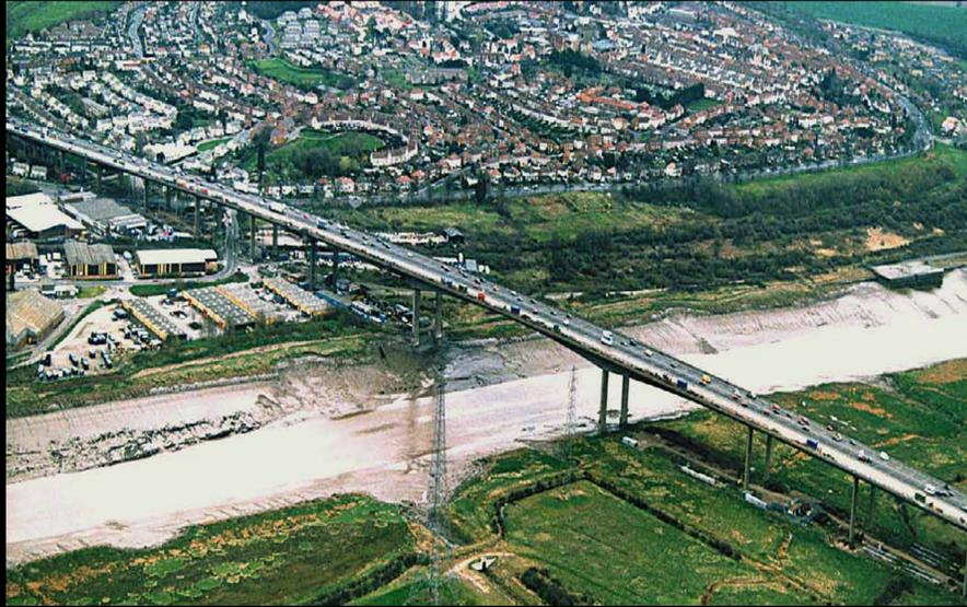
Avonmouth Bridge is a twin steel box girder bridge carrying the M5 motorway between junctions 18 and 19 just west of Bristol. It is 1.4km long, with spans from 30m to 174m. The original structure was designed to BS 153 loading and opened to traffic in 1975. Since this time loading intensities have considerably increased and highway structures are now required to carry the design loading specified in BD 37/88.
