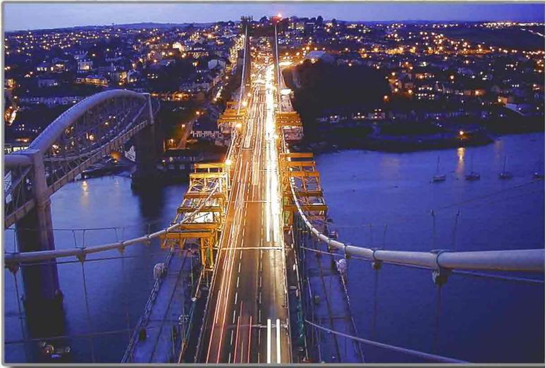
Tamar Suspension Bridge carries the A38 across the River Tamar just north of Plymouth. Opened in 1961, the 335m main span was then the longest in the UK and the structure is now the fourth longest suspension bridge after Humber, Forth and Severn. The original structure was designed to BS 153 loading and opened to traffic in 1961. Since this time loadings have considerably increased and highway structures are now required to carry the design loading specified in BD 37.
